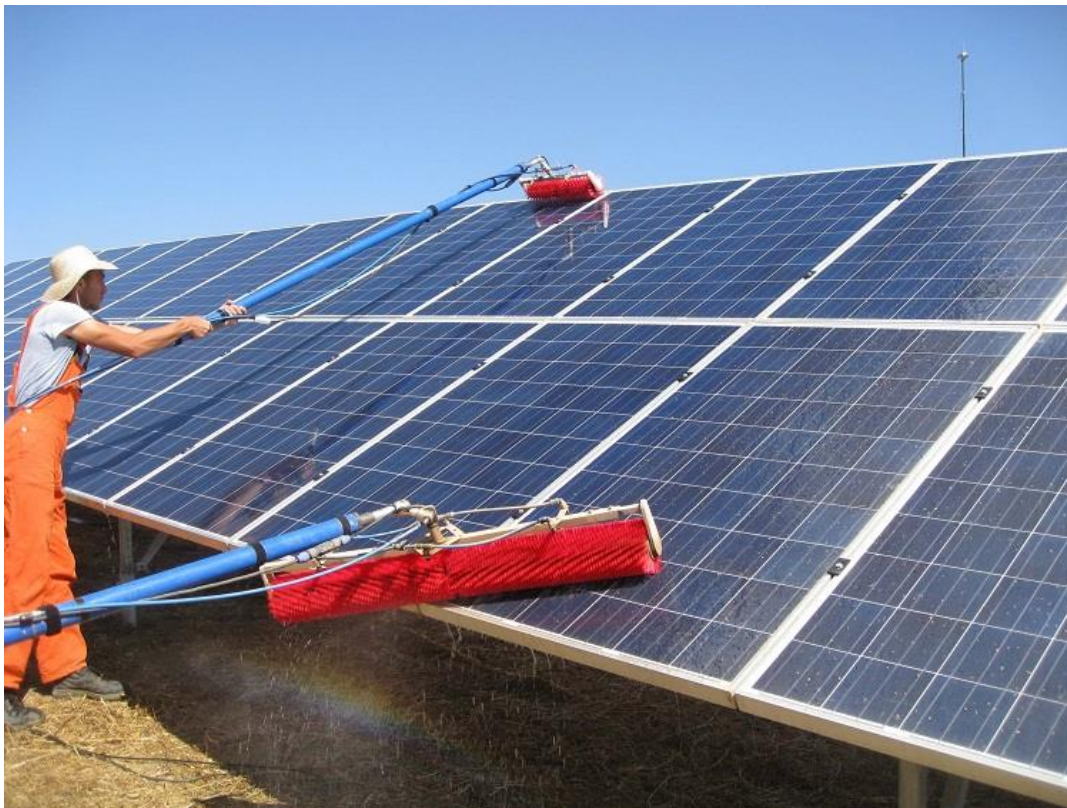
Figure 62 Manual dry cleaning of solar panels
