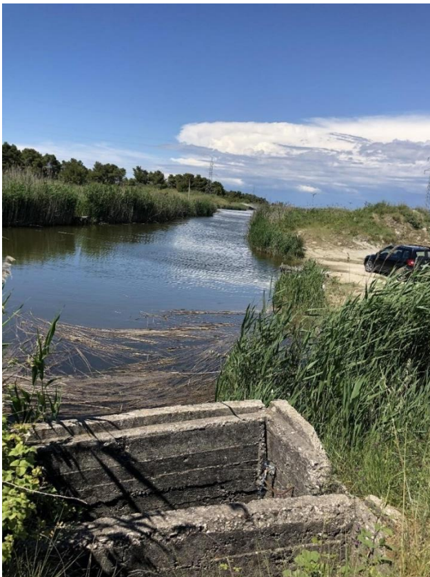
Figure 30 The drainage canal on the western boundary of the property
