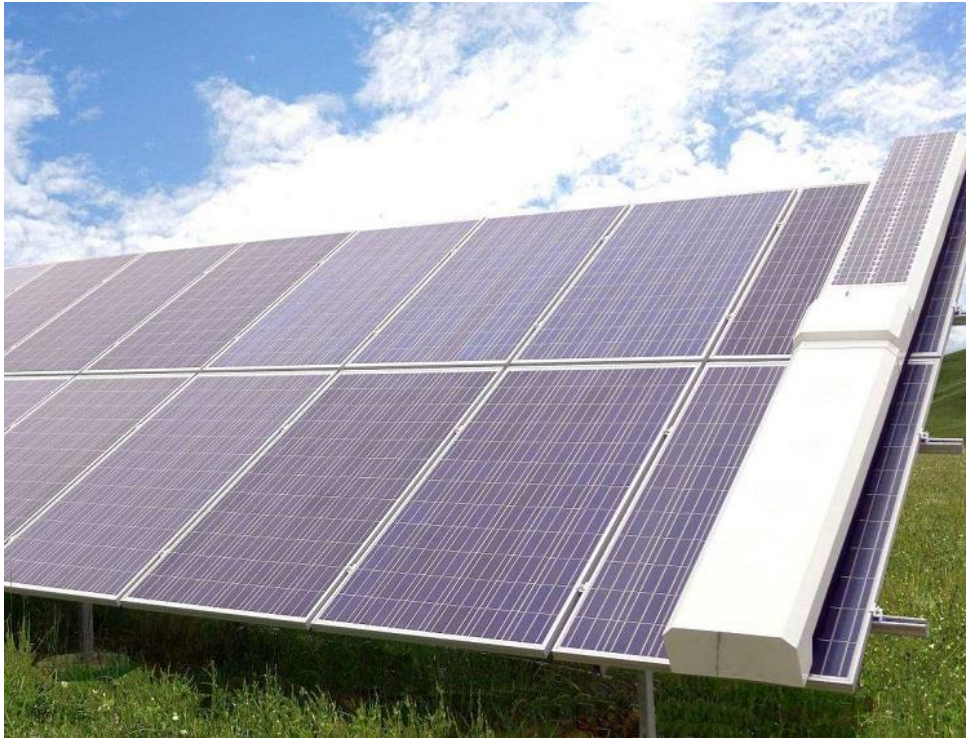
Figure 63 Robotic cleaning
