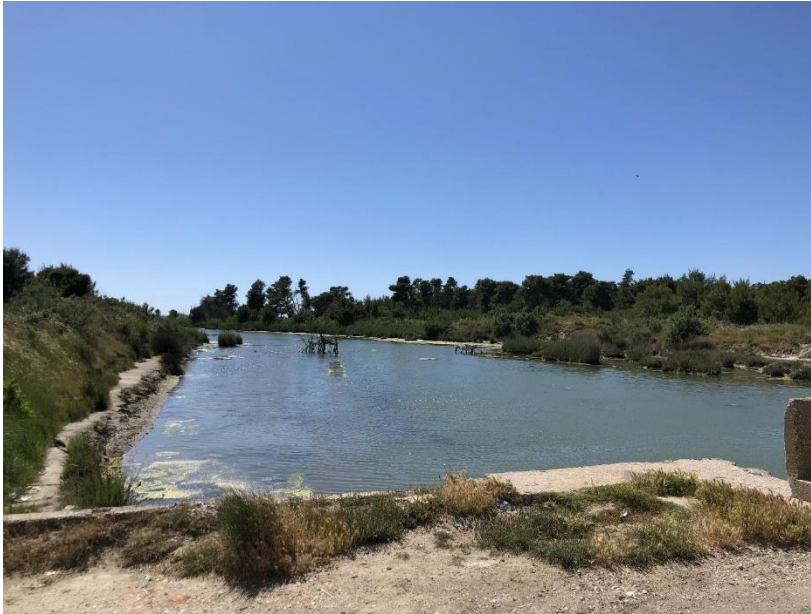
Figure 29 View of Hoxhara Pumping Station in the west of the project
